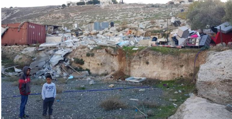
House demolition in Khalit Abed, Abu Dis
